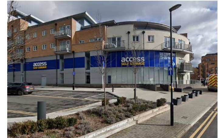
2. Woodall Court, residential co-location with B8 uses. New-build residential development at Whitestone Way.
