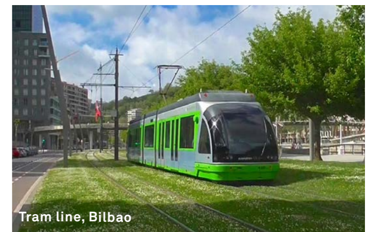
6. Urban integration of tram line into a safer environment, allowing multiple-informal crossings.
